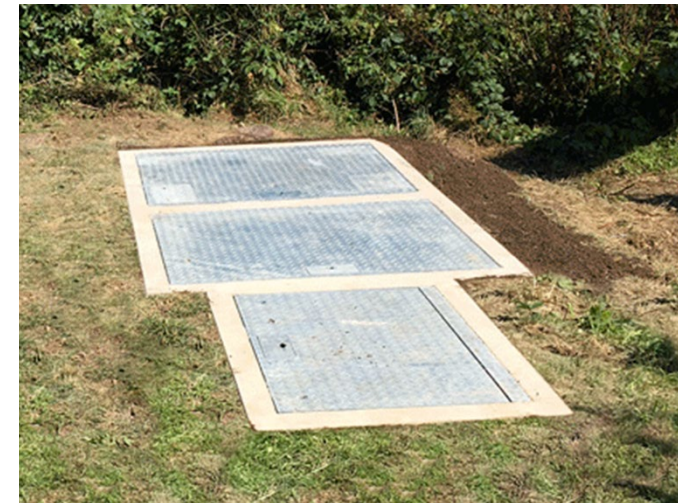
Example of typical flush covers to be used over shafts. Photo credit & acknowledgement: Technocover Limited
