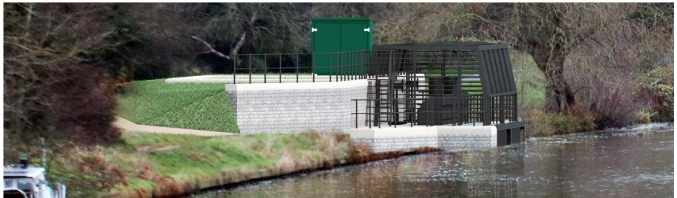
Indicative photomontage of the intake structure upstream of Teddington Weir.
