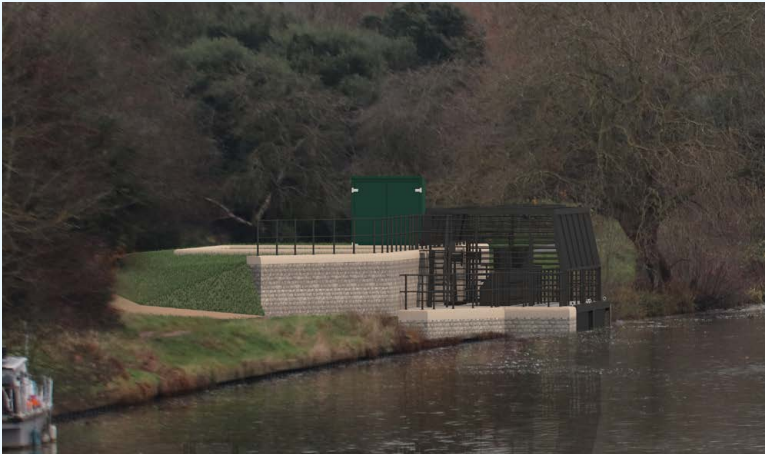
An indicative image showing the intake structure upstream of Teddington Weir
