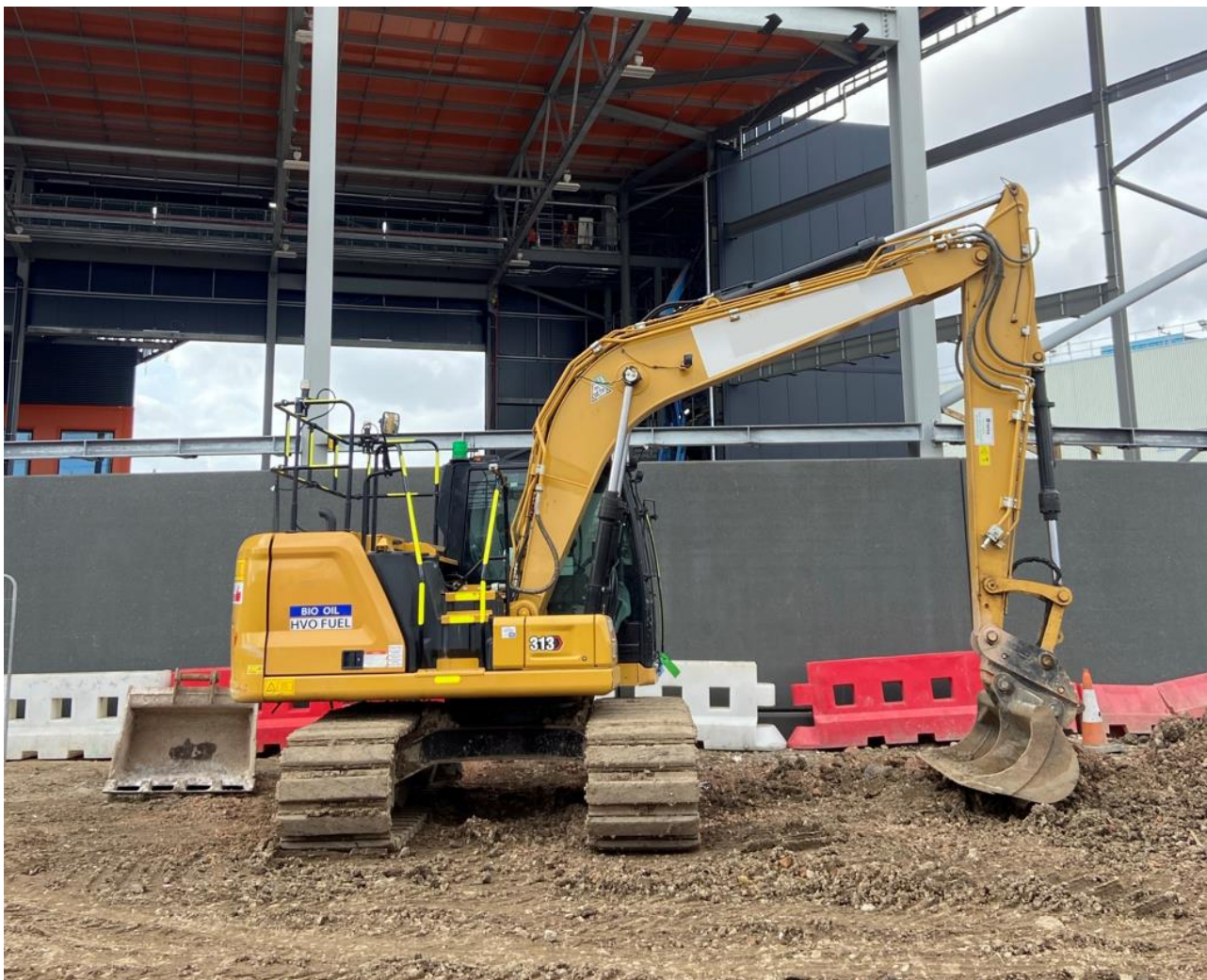
Plate 2-10 Image of a typical excavator
