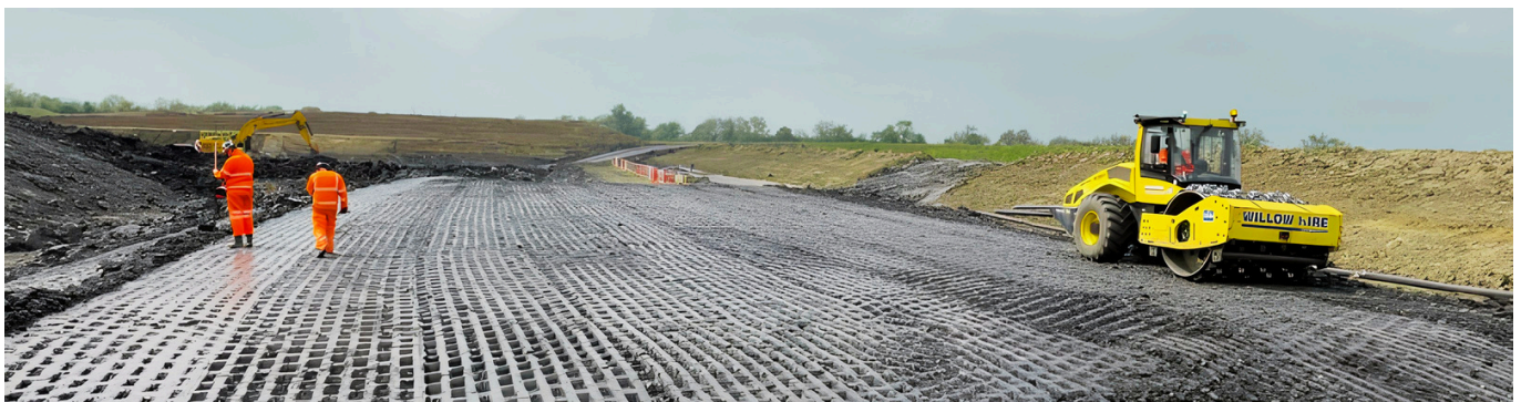
Figure 3: Compaction of Kimmeridge Clay trial panel
