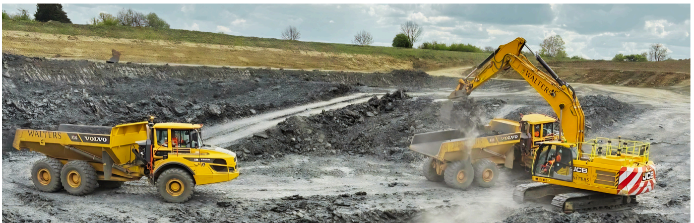
Figure 2: Excavation within borrow pit
