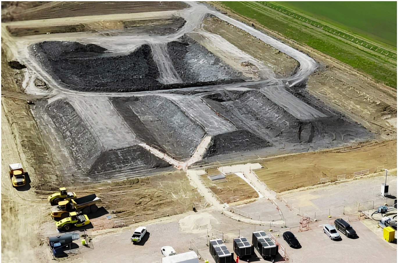
Figure 1: Aerial view of clay compaction trial
